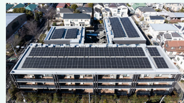
Solar panels installed across the entire rooftop
