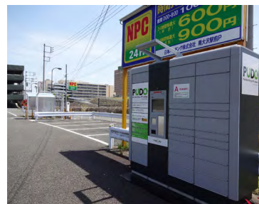
NPC24H Minami-osawa Station Front Parking (Outdoor Installation)
