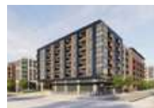
555 Herndon Parkway Project (for-rent condominiums)
