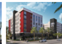
Campanile at SDSU Project (for-rent condominiums)
