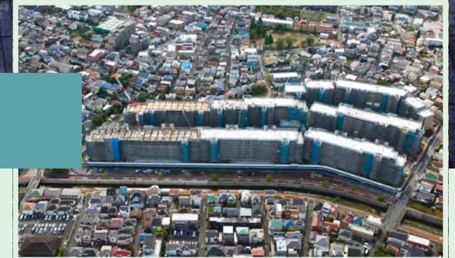
Brillia City Shakujii Koen ATLAS under construction (aerial view of site)
